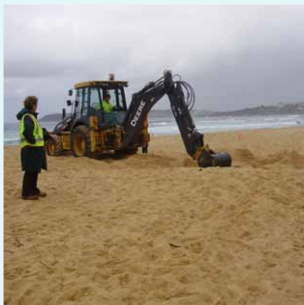
Mechanical Lagoon Opening at Curl Curl Lagoon. Source: Warringah Council.
