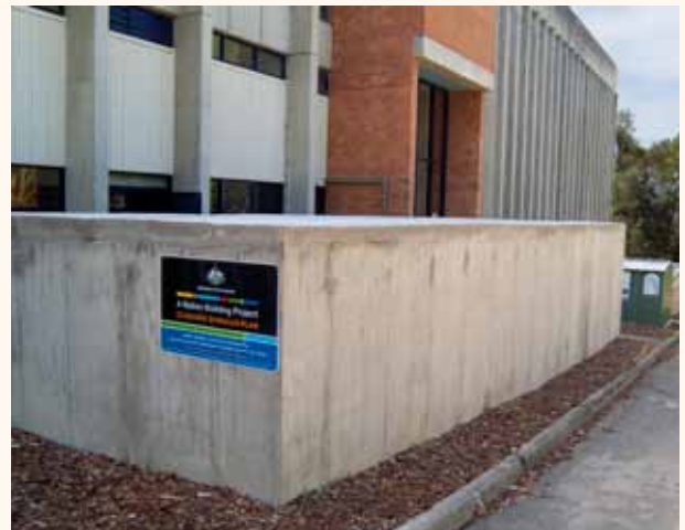
Backwash Recycling Plant - Warringah Aquatic Centre. Source: Warringah Council
