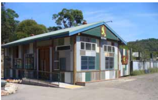
Kimbriki Eco House. Source: Warringah Council
