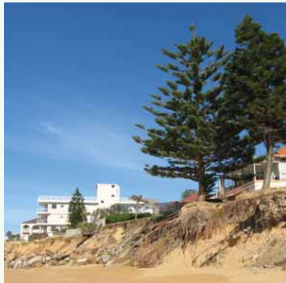
Narrabeen Beach storm damage June 2007. Source: Warringah Council
