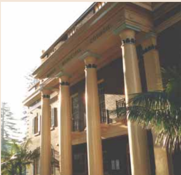
Manly Council Civic Building. Source: Manly Council
