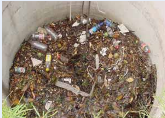
Pollutants captured by the SQID, improving water quality. Source: Mosman Council
